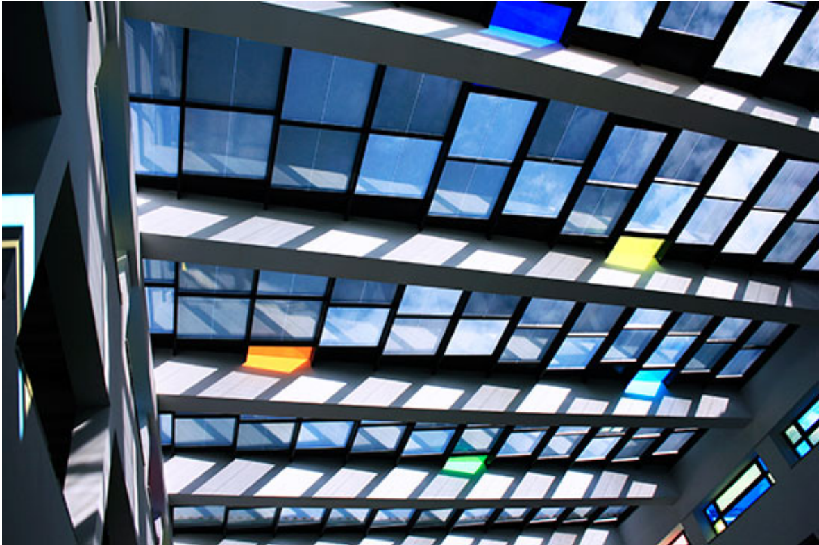
Bejar Markt, Salamanca (ES), transparente Photovoltaikanlage der Dachverglasung, Photo Copyright by Onyx Solar
