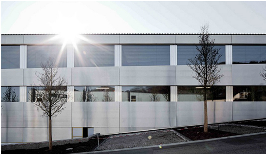
List Customer Centre Arisdorf, Switzerland, Christ & Gantenbein AG Architekten ETH SIA BSA 2015
